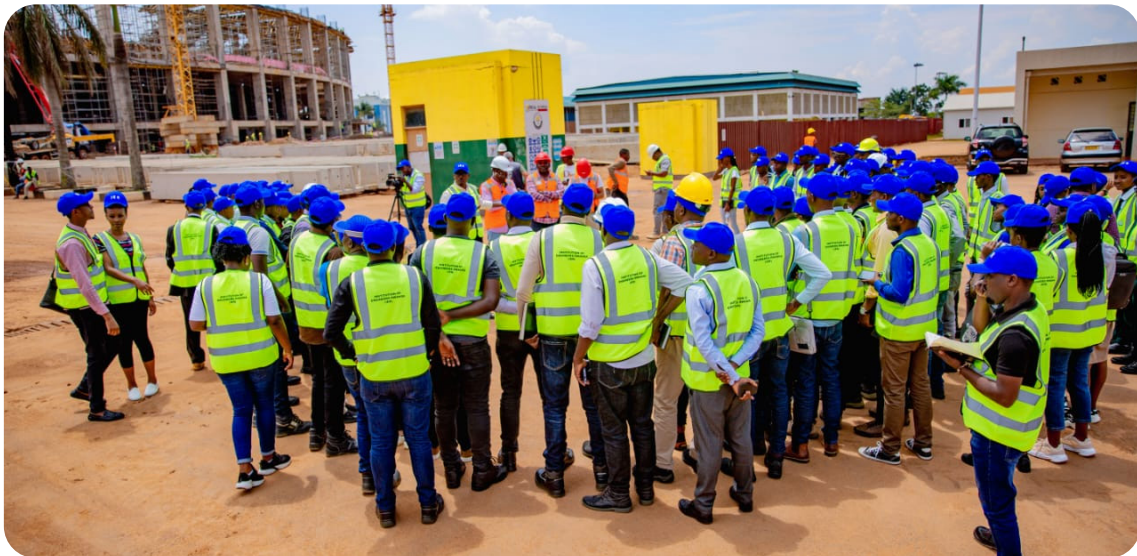
IER team visiting ongoing works at Amahoro stadium renovation works
